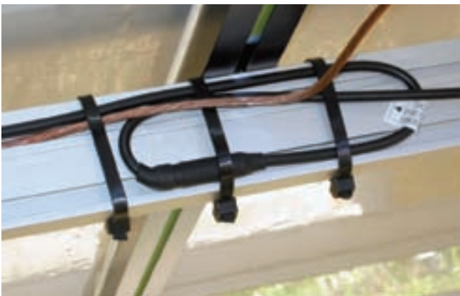
Above: Black UV-resistant cable ties used to secure array wiring. At right: Stainless steel "loop clamp" and hardware.
