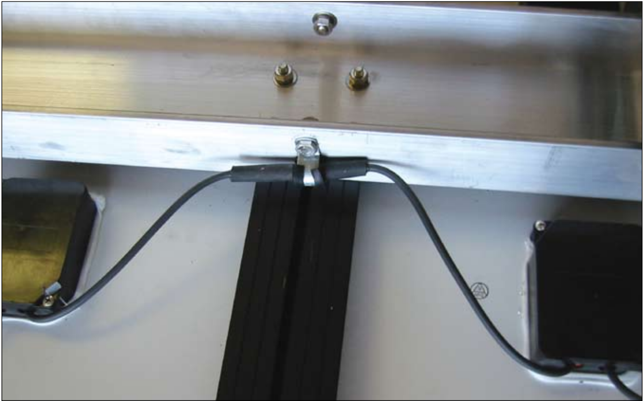
Photo 5. Shortened, spliced, and secured module interconnections
