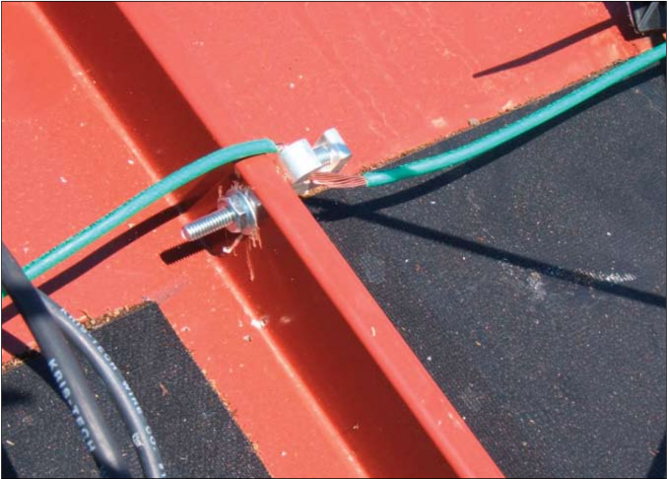
Photo 6. Grounding a metal roof, THHN questionable
