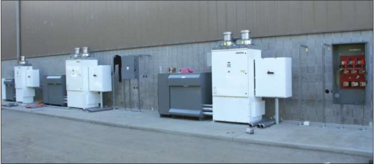
Photo 3. 250 kW inverters
