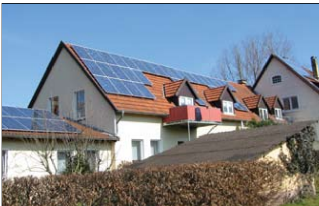
Photo 4. Residential rooftop PV array
