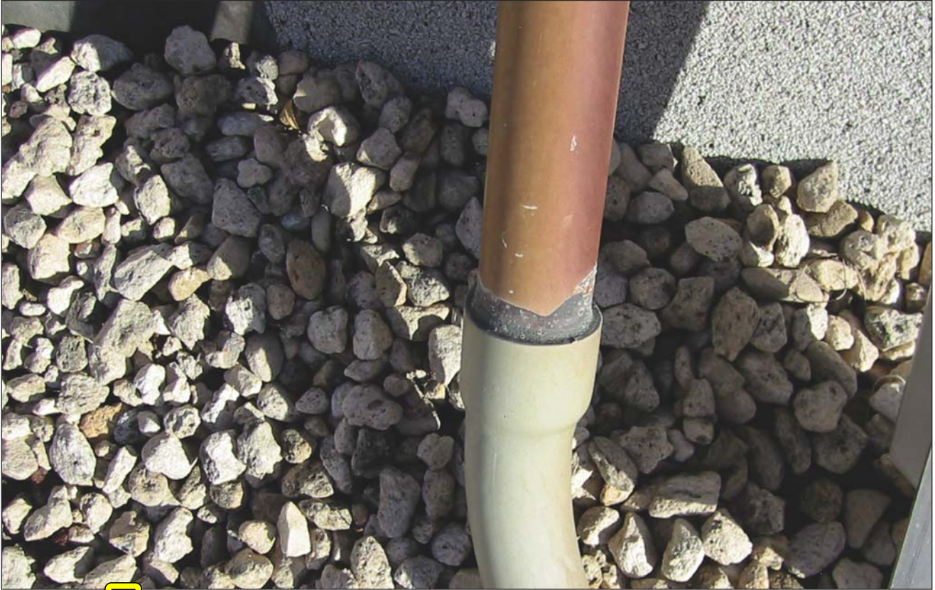
Photo 3. PVC conductor, darkened with age
