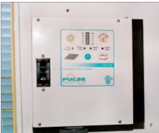
Photo 7. 60 A PV charge controller
