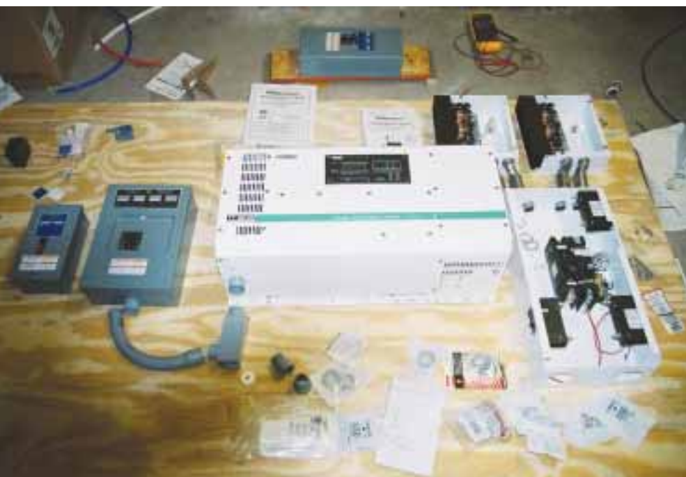
Laying out the energy conversion equipment.
