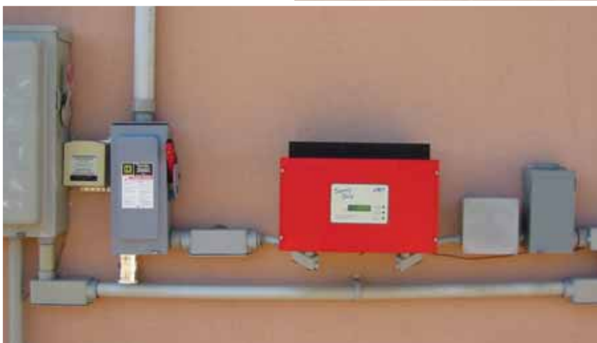
Figure 1. Utility-interactive inverter
