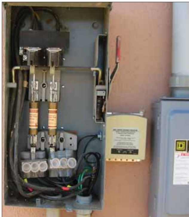
Figure 3. PV inverter output connected to service conductors
